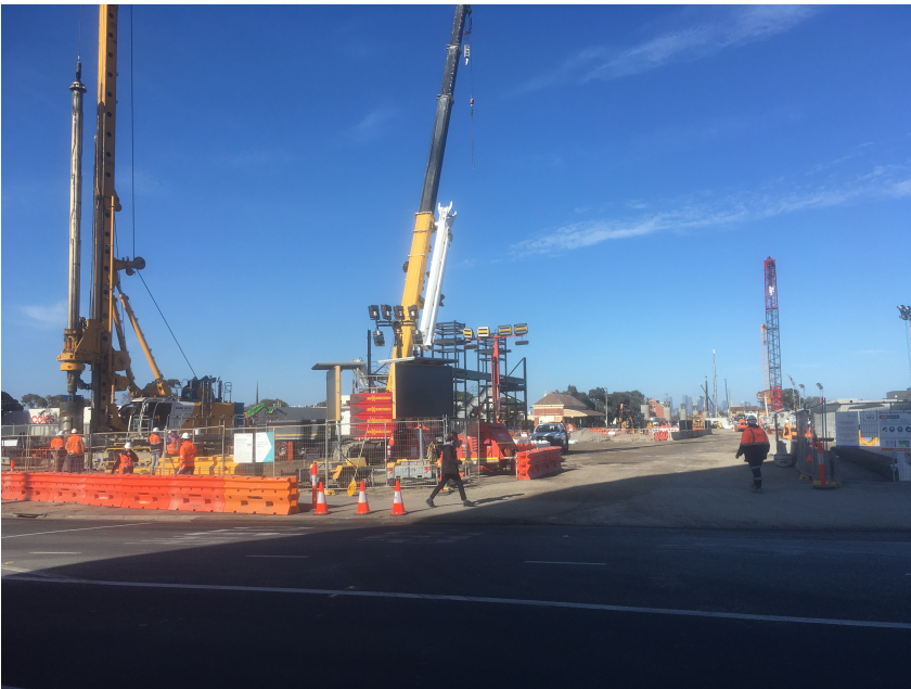
Some photos of the Upfield line level crossing removal works, looking south towards Bell Street from around Batman station.
