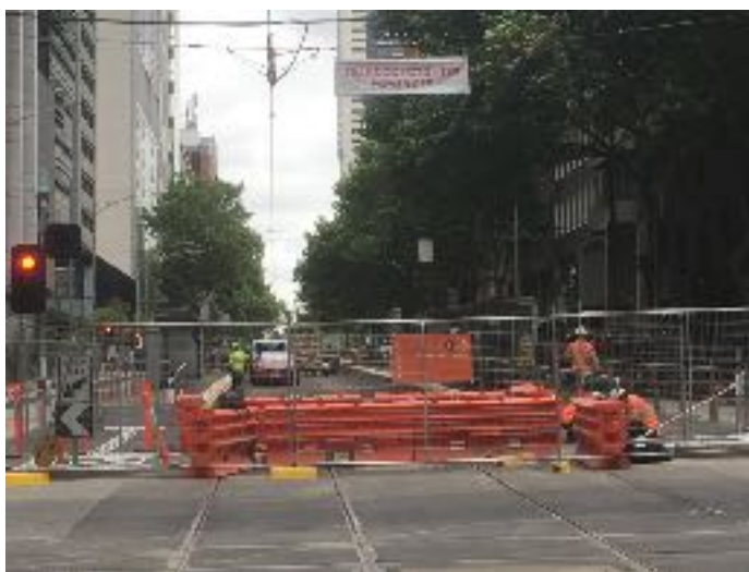
Works in William Street
