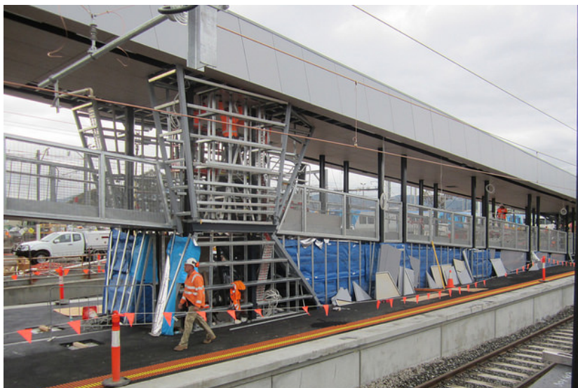
Level crossing removal works at Bayswater station - photo from Daniel Bowen
