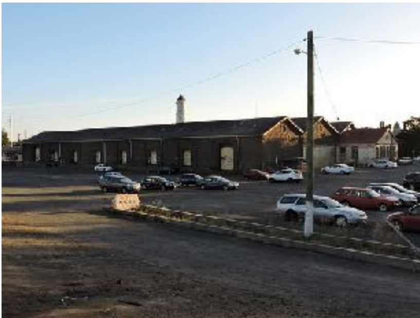
The bluestone good sheds at Ballarat station. Photo from Ben Lever
