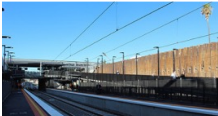
The new Bentleigh station (photo from Daniel Bowen)
