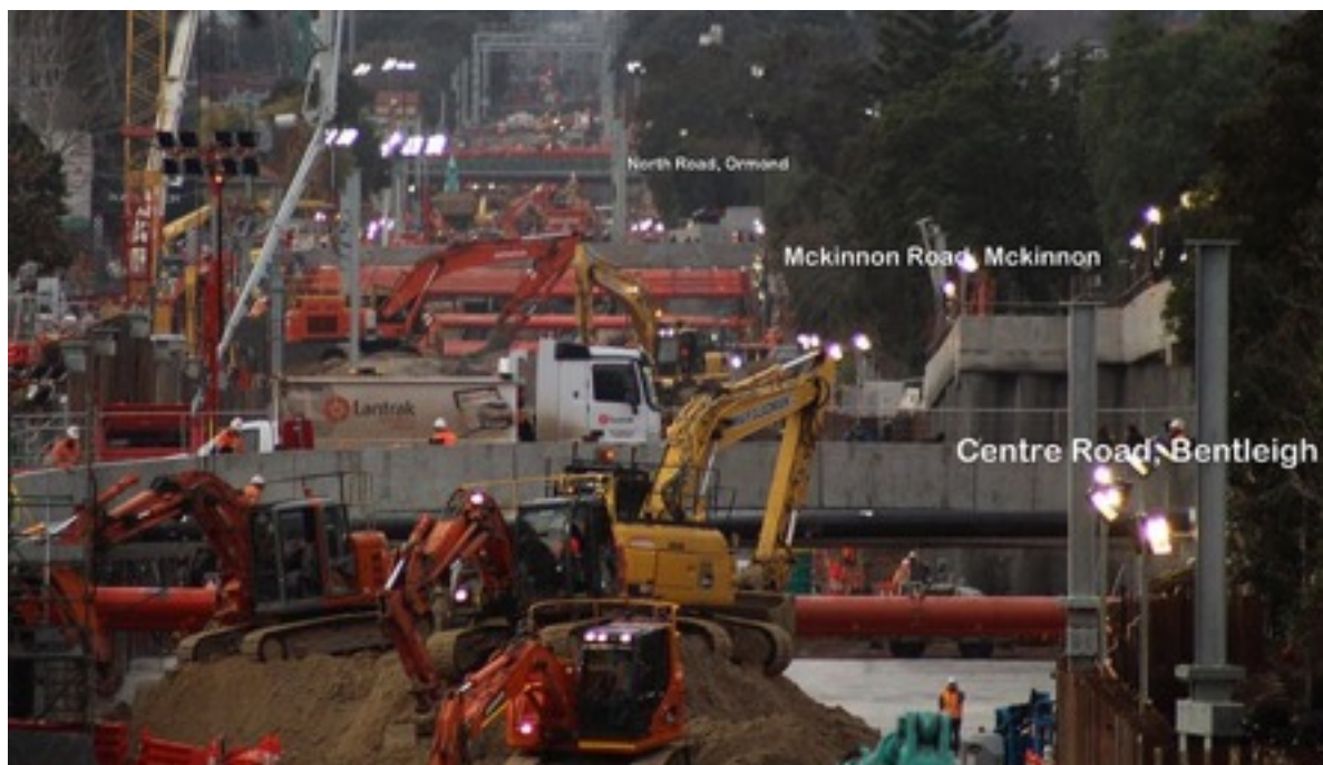
Level crossing removal works on the Frankston line.
