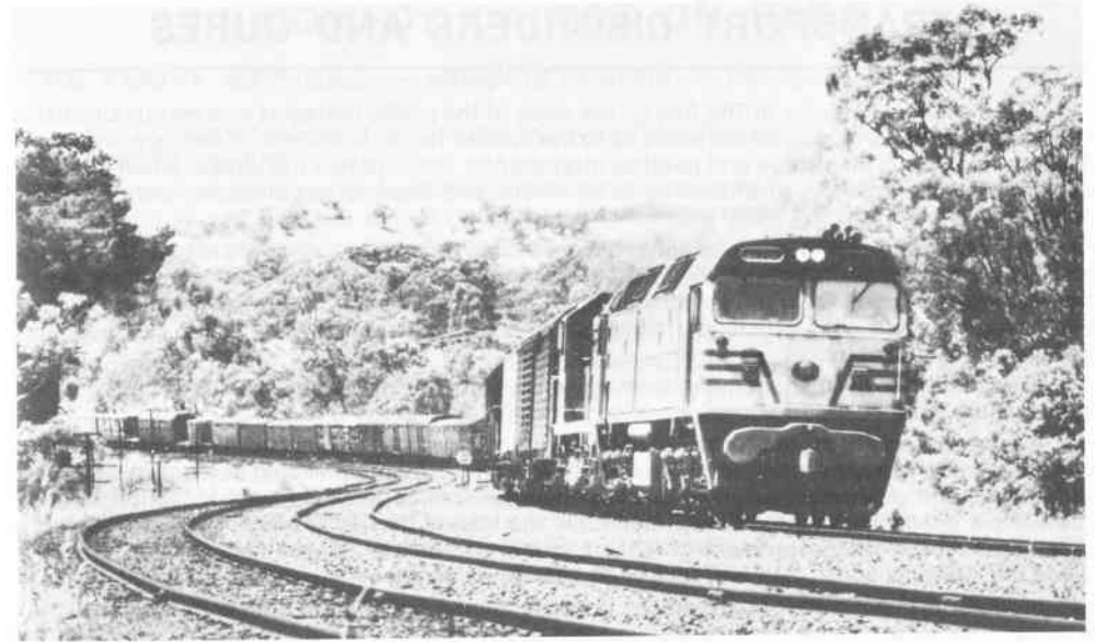
Broadford curves: Examine closely the broad gauge curves showing unevenness & erratic elevation (the train is on the standard gauge track). Text, table and photograph are courtesy of Newsrail
