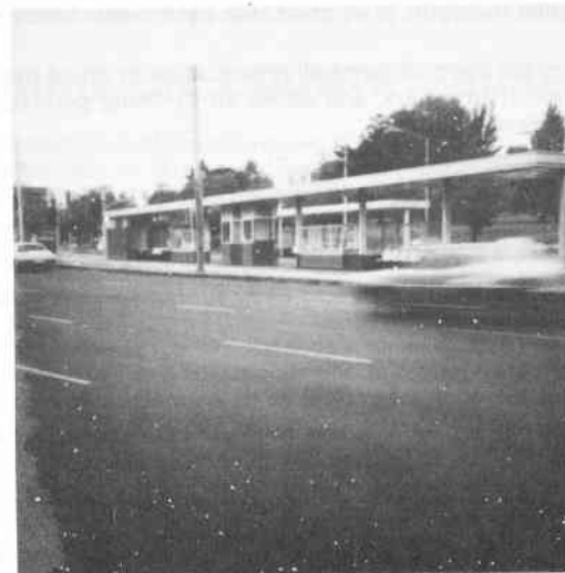
The new transport interchange at Domain & St Kilda Roads, opened on 17th November.
